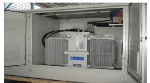
Less-flammable Liquid Type (Silicone fluid)
