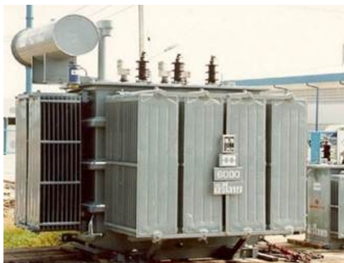
Open type conservator tank
